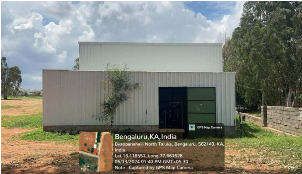
Fig 3: STP for waste water recycling
